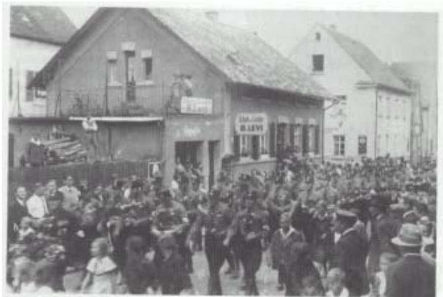
20 metres in front of the Dottheim-House in 1935
